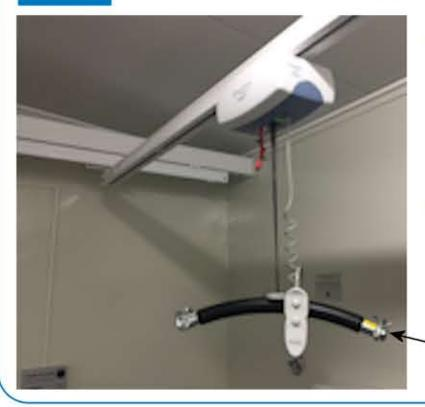
Charge Indicator Hand Control Cord Hold and use the spreader bar to pull the hoist into a clear area for safe use. Make sure there are no obstructions around you
